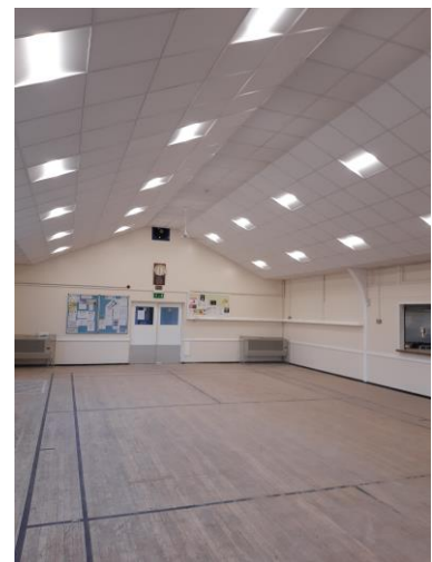
Pictures above show the new suspended ceiling being installed and the integrated lighting
