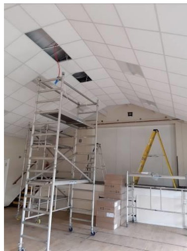
Pictures above show the new suspended ceiling being installed and the integrated lighting
