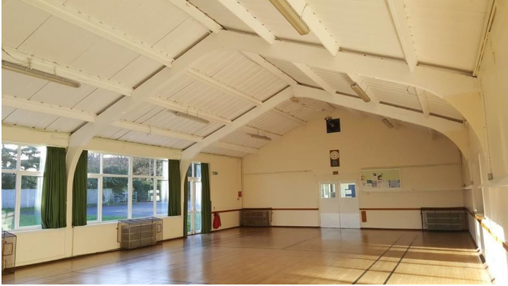
The main hall before refurbishment works.
