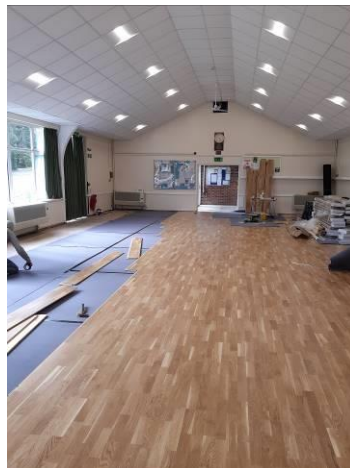
New floor being installed
