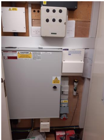
Replaced and upgraded electrical mains switch gear
