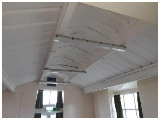
Replacement back hall LED strip lighting
