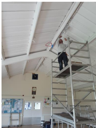
Pictures above show the new suspended ceiling being installed and the integrated lighting
